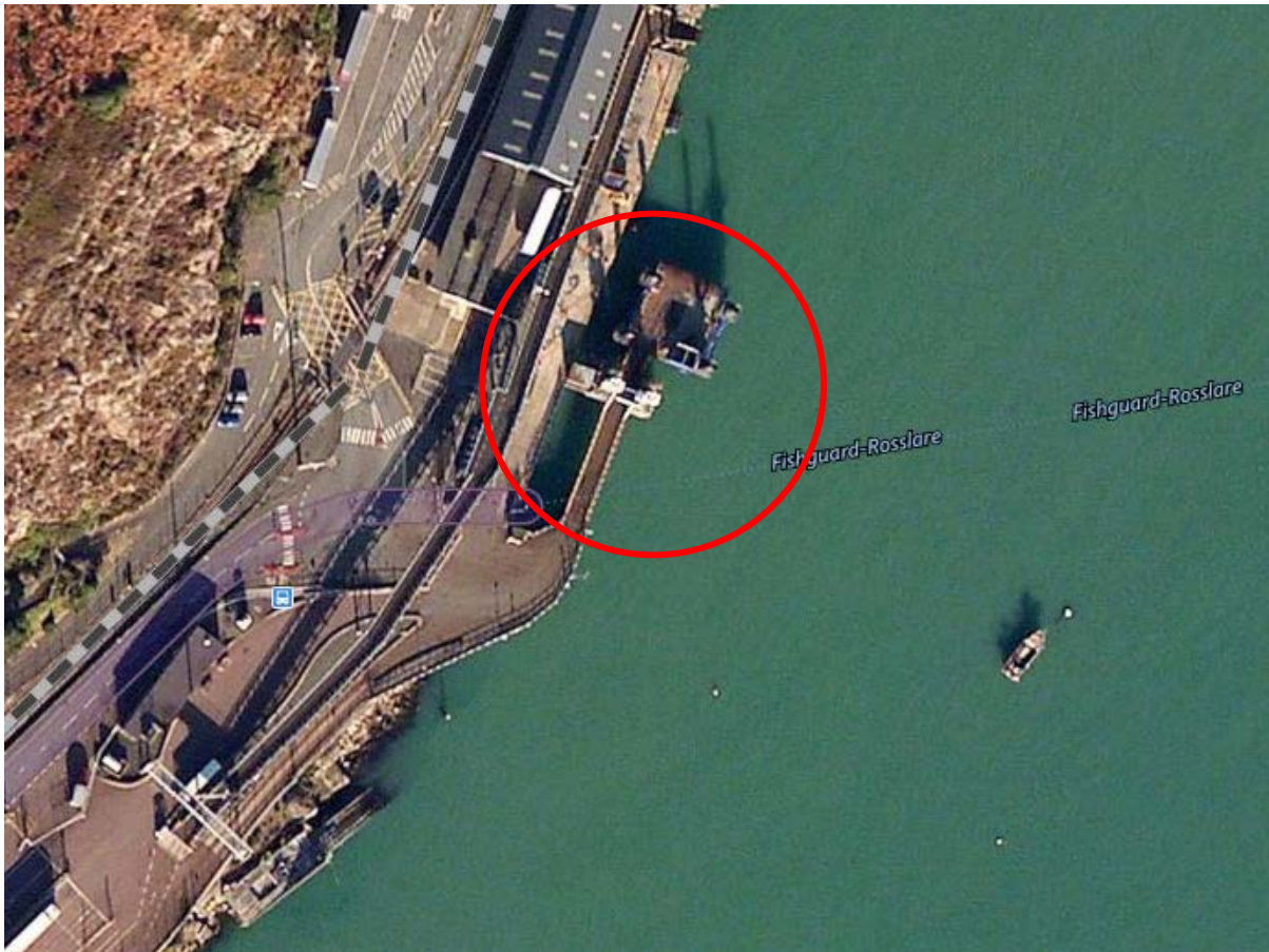
Figure 16.3 Existing Linkspan Location
