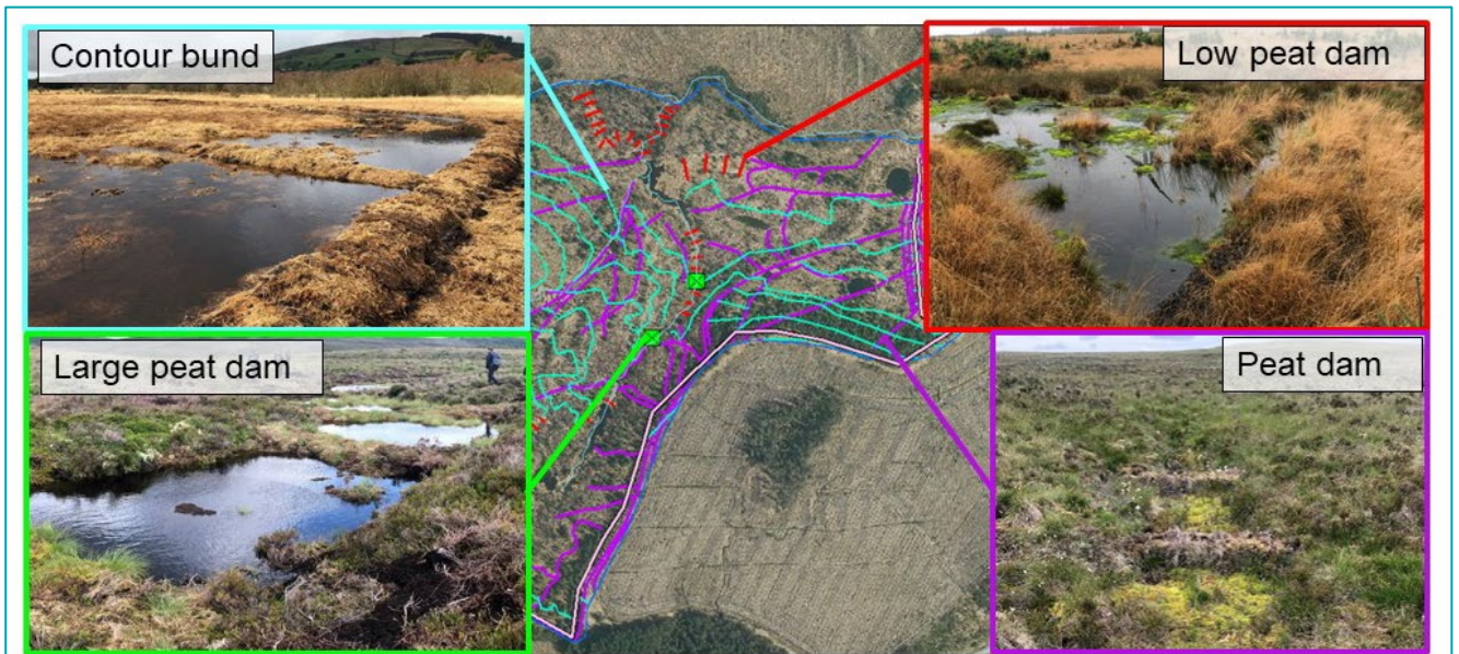
Figure 8. Restoration design incorporates multiple features, such as dams and contour bunds in hydrological management to optimise the restoration potential of the peatland.
